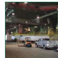
GTS begins renovation to make facility more efficient and cost-effective
